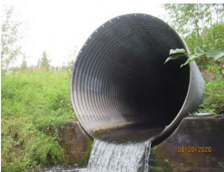
Spring Creek Drive Culvert— Fair Condition
