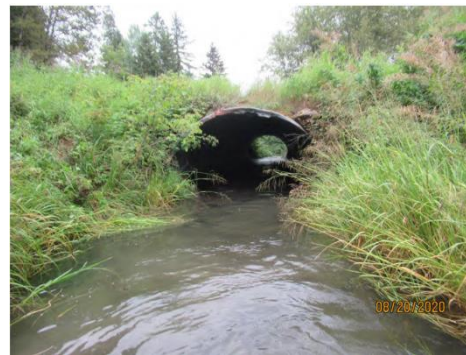
Meadow Brooke Lane Culvert— Good Condition
