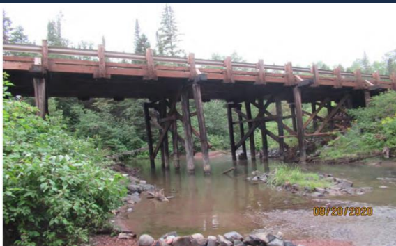
Cold Water Bridge— Fair Condition
